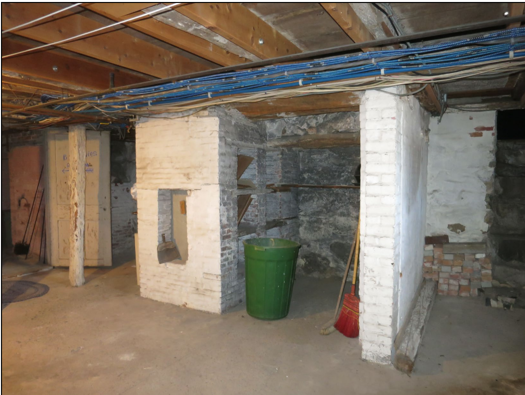
Basement, east side showing base for hearth and oven in SE front room.
