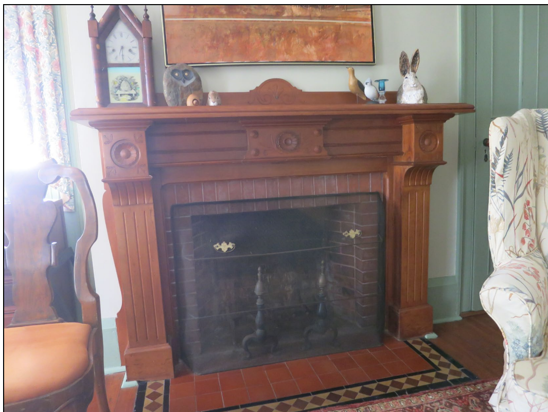
First floor, SW front room, detail of fireplace, mantel & hearth added ca. 1907.
