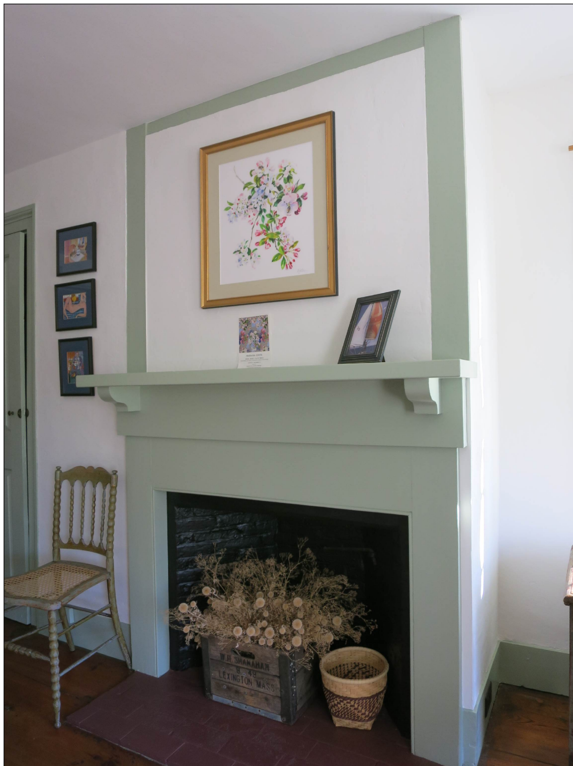
Second floor, SE chamber, detail of fireplace with added shelf.
