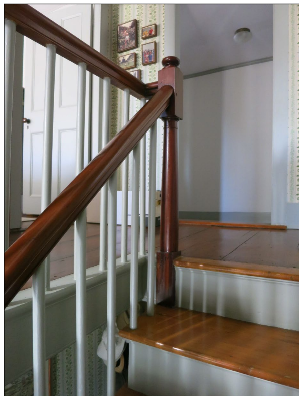
Second floor, detail of railing.
