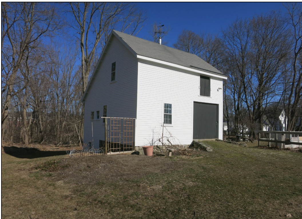
View of barn from SW.
